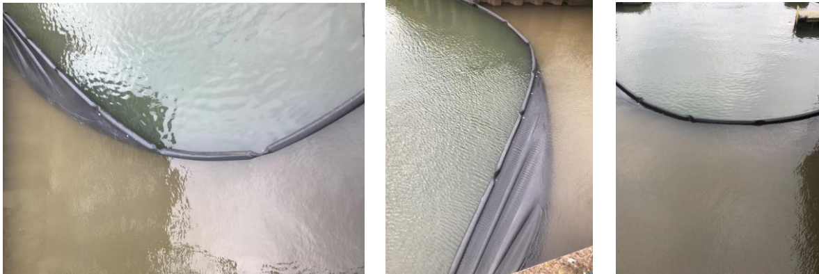
Figure 4.1: Photos demonstrating silt curtain at Exmouth Marina entrance during dredge operations (Source: Lewington and Irwin, 2018)
